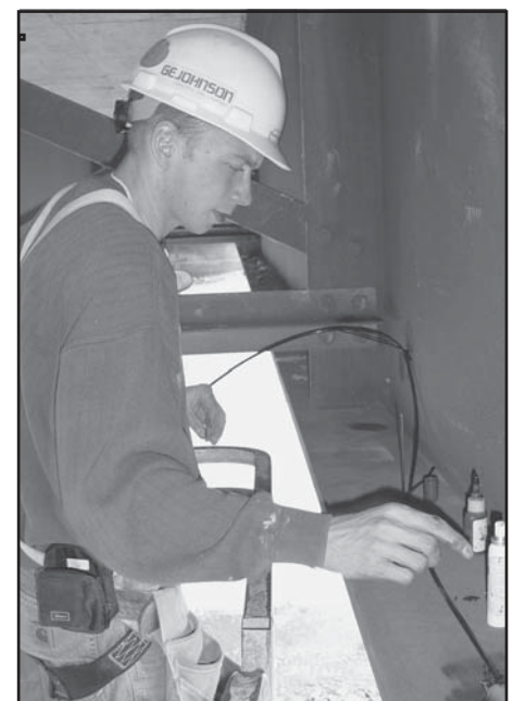
Graduate student Derek Hemphill prepares the bridge for continuous remote monitoring.
