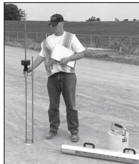
Figure 3. Operating dynamic cone penetrometer
